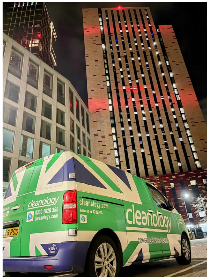
Cleanology's brand new offices in London's new skyscraper district of Vauxhall Nine Elms
